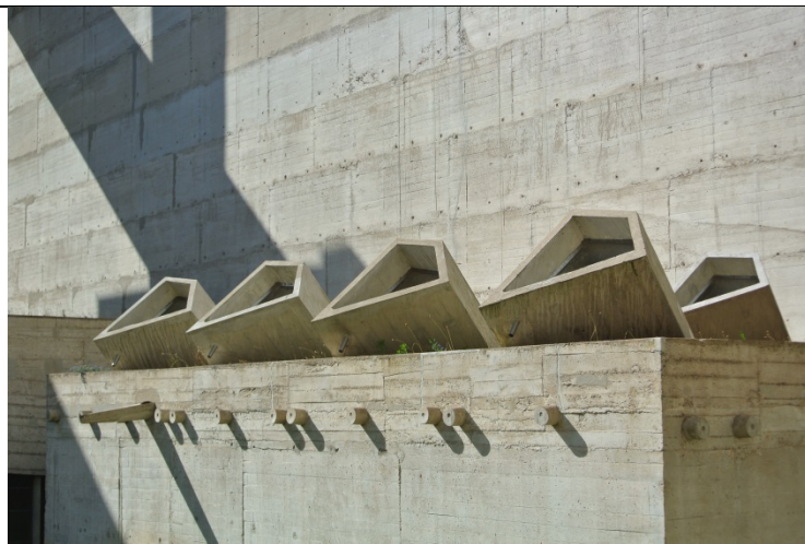
15 – Lucernarios Convento La Tourette – Le Corbusier
