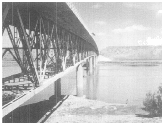
Bridge over the Santa Cruz river. Present photograph.
