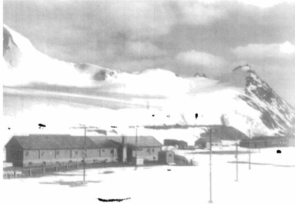
Meteorological and geomagnetic observatory of Laurie Island in Orcadas del Sur.
